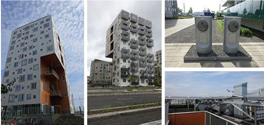
Fig. 2 Det Store Havnehus—view on both facades, recycling bins outside the building, solar installation on the roof. Photographs M. Mokrzecka
